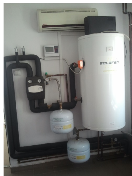
Figure 7. Pump and boiler connected to the thermosolar panels
